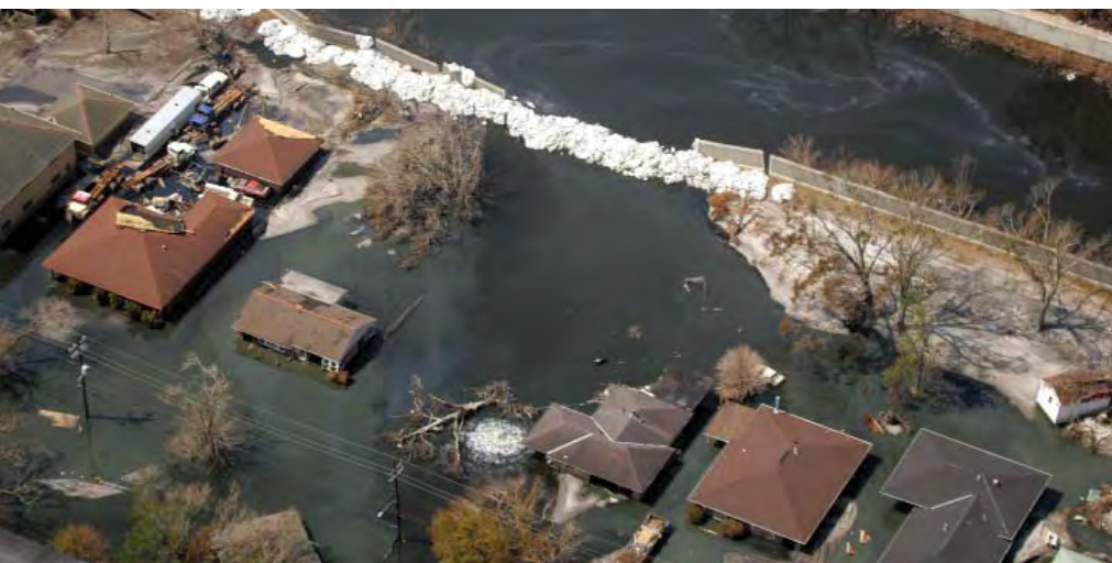
One of the levees that broke, releasing flood waters into residential neighborhoods.
